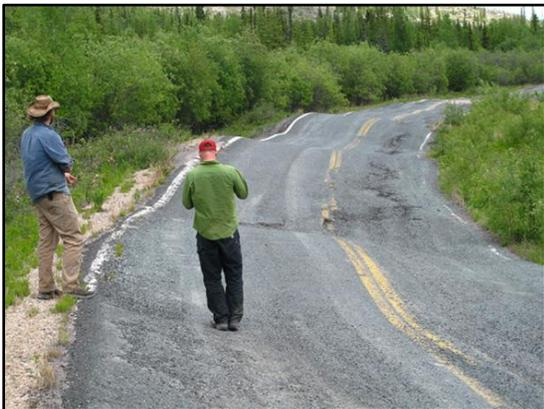
Figure 6. Abandoned section of Highway 4, east of Yellowknife. The paved road surface has continued to settle due to permafrost thaw after it was abandoned in 1999.
